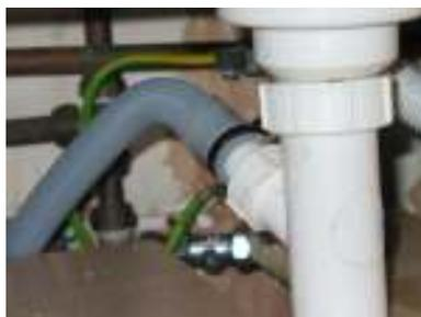
Sometimes the drain hose will be into a stand pipe. If this is the case this will not be causing the problem. If the stand pipe was blocked it would leak.
