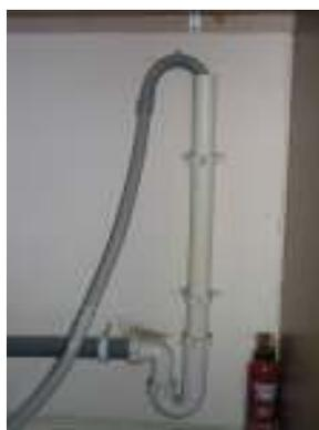
If the drain hose is not long enough, it is easily extendable with a kit. If fitted into a stand pipe, cable tie into position so it does not 'jump out' as you push the machine back. If fitted to sink waste, fit to the sink waste and use a clip if needed to secure, and then check for leaks.
